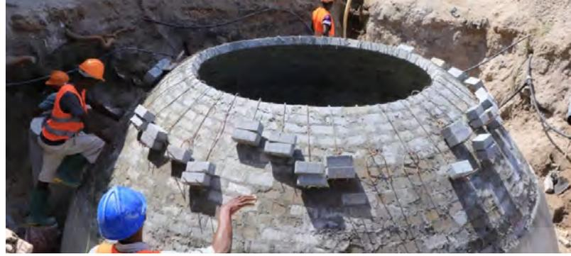
*Biogas digesters, like this one under construction at Mwananyamala Hospital in Tanzania, allow for the safe disposal of food waste and placentas, while generating biogas for use at the facility*
